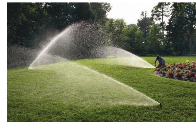
Rain Bird 5000 series sprinkler for ornamental landscaped areas of the course
